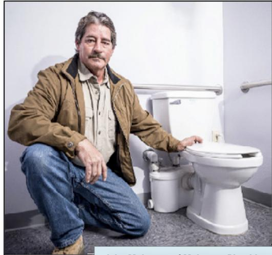
**John Mulvaney of Mulvaney Plumbing Systems with the Sanibest Pro macerating system he installed at Hajoca Orlando. With the Sanibest Pro, Mulvaney had the new customer restroom "up and running in a day," says manager Jim Holtzapple.**
