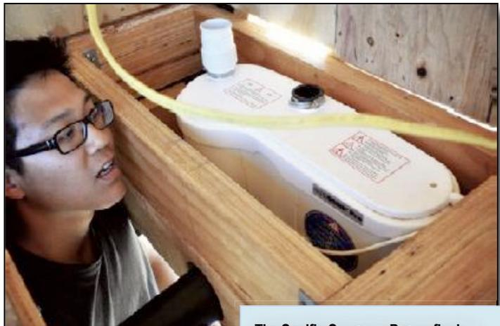
The Saniflo SANIGRIND PRO upflush grinder system is installed beneath the floor in the SCI-Arc/Caltech team's net-zero home for the 2013 Solar Decathlon competition in Irvine, Calif.
