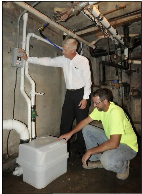
Don Smith of Irr Supply (left) with Scott Kuhns of RIC Plumbing of Lockport, N.Y. Although it was his first Sanicubic installation, Kuhns finished his work in just one day. "This pump is well-suited for the application. The building is very old and digging would have been very difficult."
