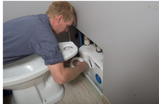
The Sanibest Pro heavy-duty grinding system (shown in wall), handles the accidental flushing of larger sanitary articles and other items a conventional plumbing system might struggle to handle.
