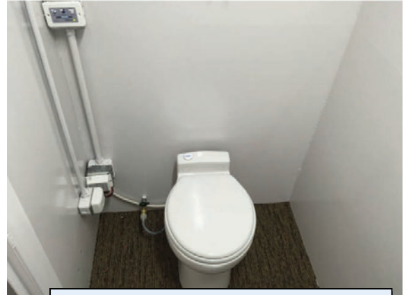
Saniflo macerating toilets grind waste to slurry before pumping it to a septic tank or city sewer, when used as part of an underground bunker.
