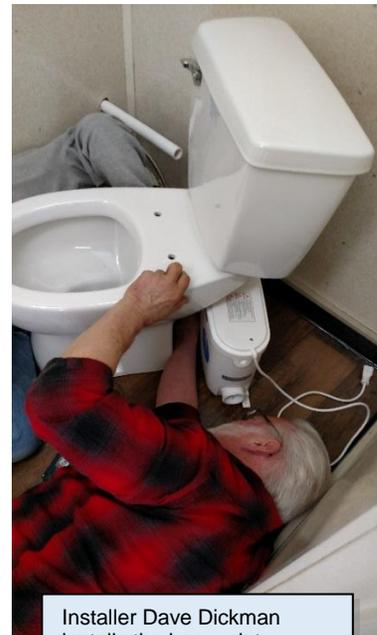
Installer Dave Dickman installs the heavy duty Sanibest Pro grinding system from Saniflo.
