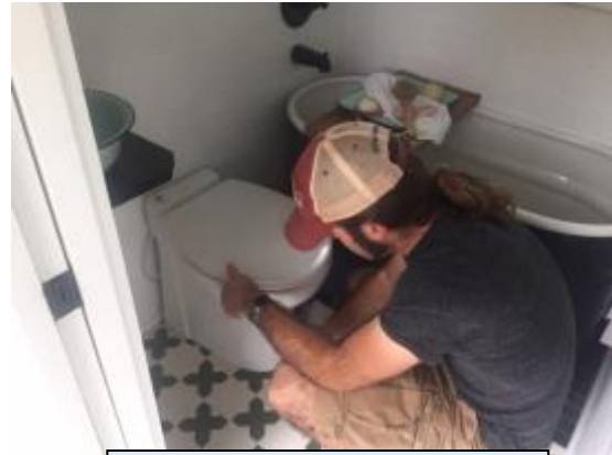
Plumbing contractor Garrett O’Neal installs the Sanicompact macerating toilet from Saniflo.
