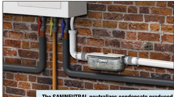
The SANINEUTRAL neutralizes condensate produced by many modern, high-efficiency appliances, preventing pipe corrosion and other lasting damage.
