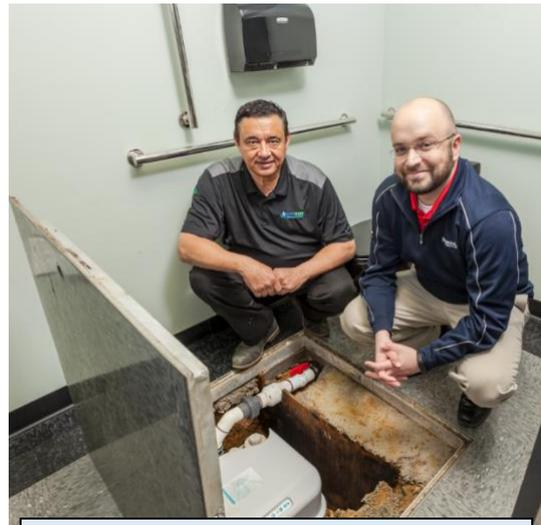
Dale Nichols of PipeTech Plumbing Technologies (left) and Nathan Smith, Ferguson Branch Manager in Raleigh, stand over the Sanicubic 2 duplex grinding system from Saniflo, which grinds and pumps effluent to the drain line.
